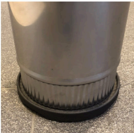
Flue seated correctly.
